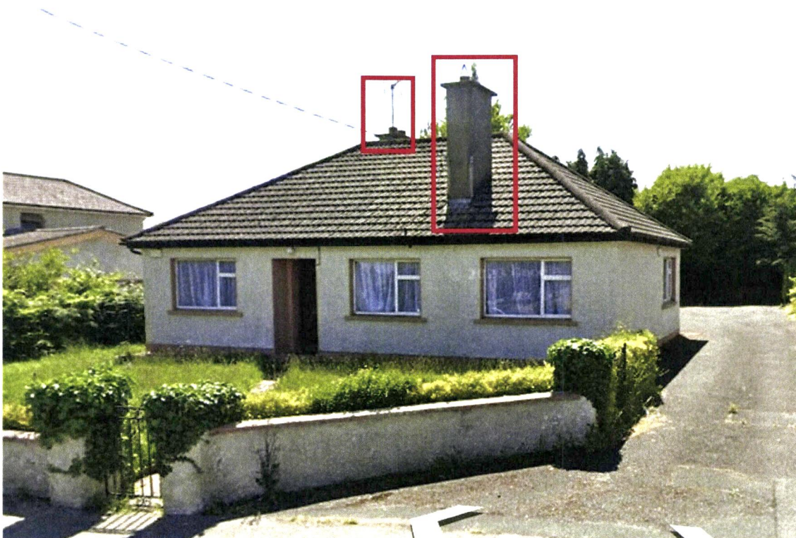
Front View: Removal of chimney
